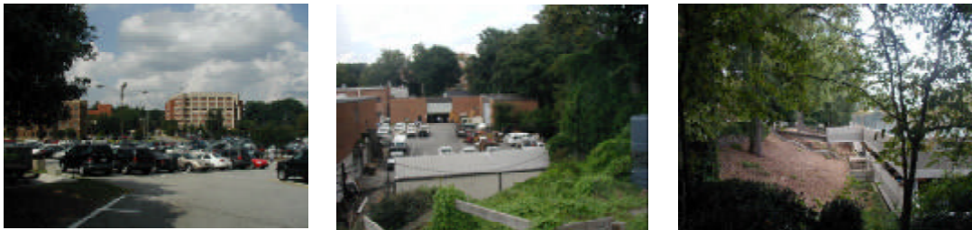
Figure 18 Required Demolition for the Eco-Commons; L-R: Parking west of Hemphill, Physical Plant, and the Peters Parking Deck.
