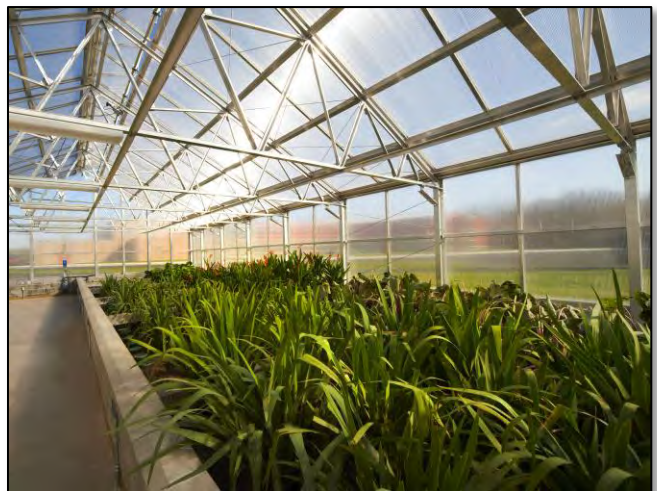
Figure 1: Inside Enclosed Ecological Treatment System
