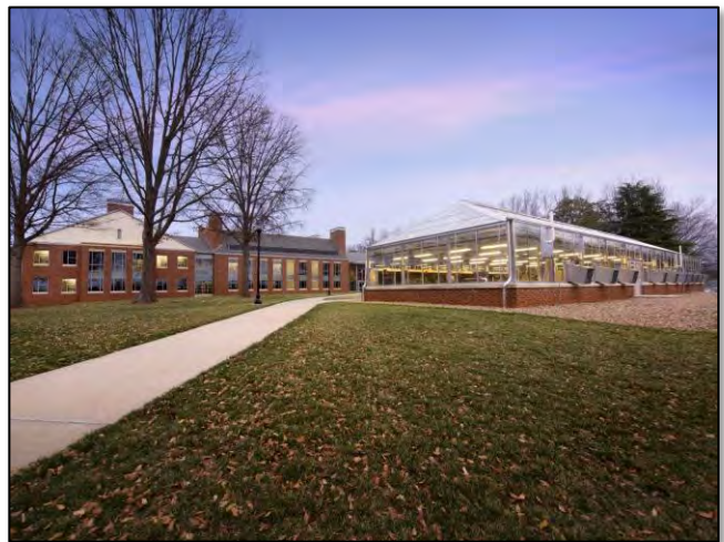
Figure 2: Exterior of Enclosed Ecological Treatment System
