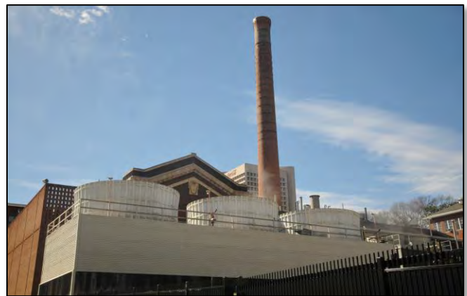
Figure 12: Holland Utility Plant
