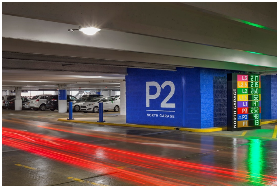
Figure 43: Parking Wayfinding and Guidance System
