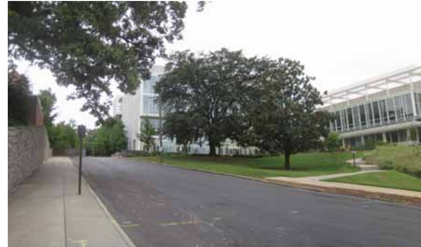
Unimproved Atlantic Promenade at Marcus Nanotechnology Building
