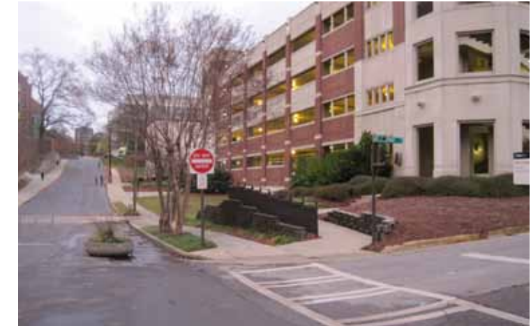
ADA access to the parking deck, looking south
