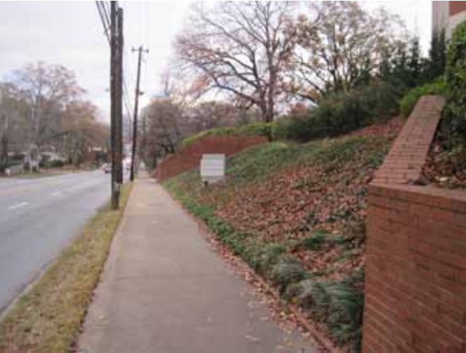
Existing 10th Street edge conditions at CRB
