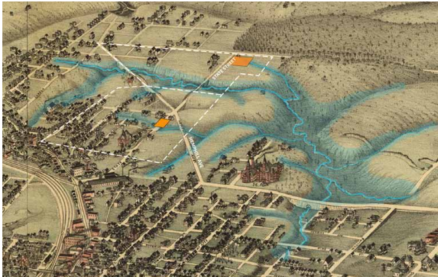
1892 Aerial View showing historic drainage patterns and limits of the Sector Plan. Orange indicates major building projects in these two sectors.
