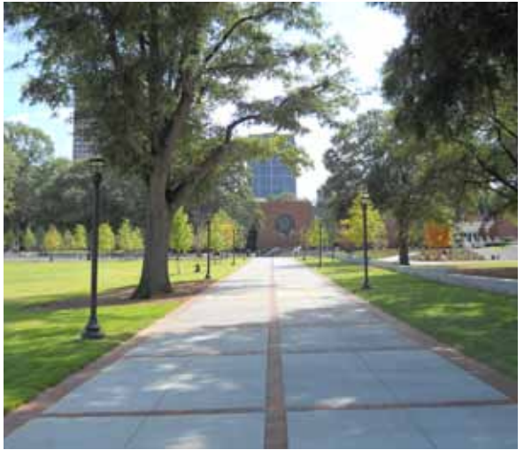
15'-20' Eco-Commons Ribbon Path - differentiate bicycle and pedestrian circulation, use pervious pavement when possible.
