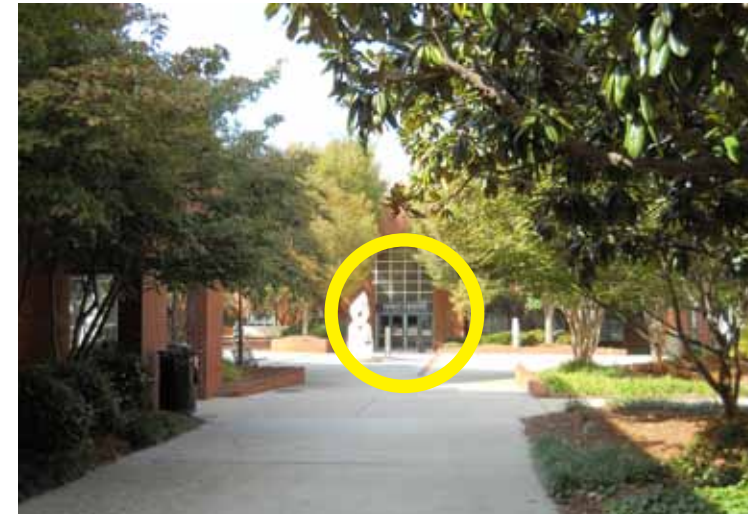
Ferst Center's primary entrance from south lacks visibility
