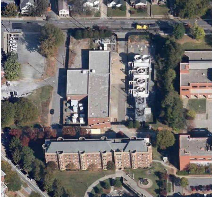
Existing chiller plant slated for expansion
