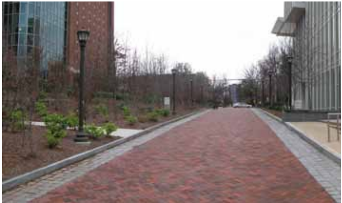
Atlantic Promenade - LMP detail 'A' - brick pavement with cobble edging
