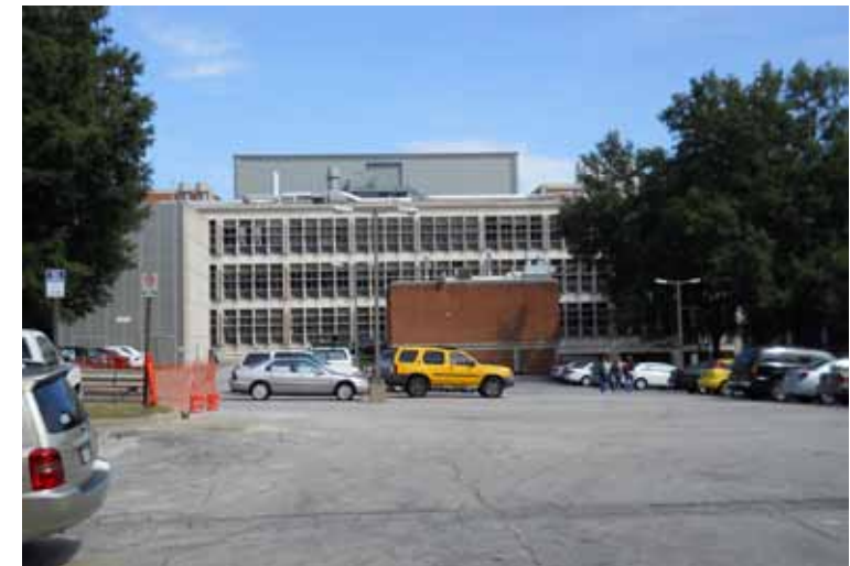
Pedestrian access to Tech Green from north crosses multiple parking lots
