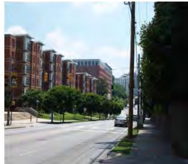
Looking east on 10th Street past the existing retaining wall
