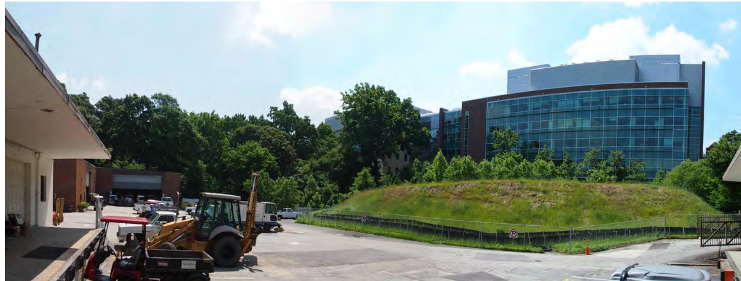
Existing view southeast towards the existing MSE building and overlook
