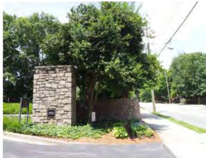
Existing rubble pier at the President's house entry
