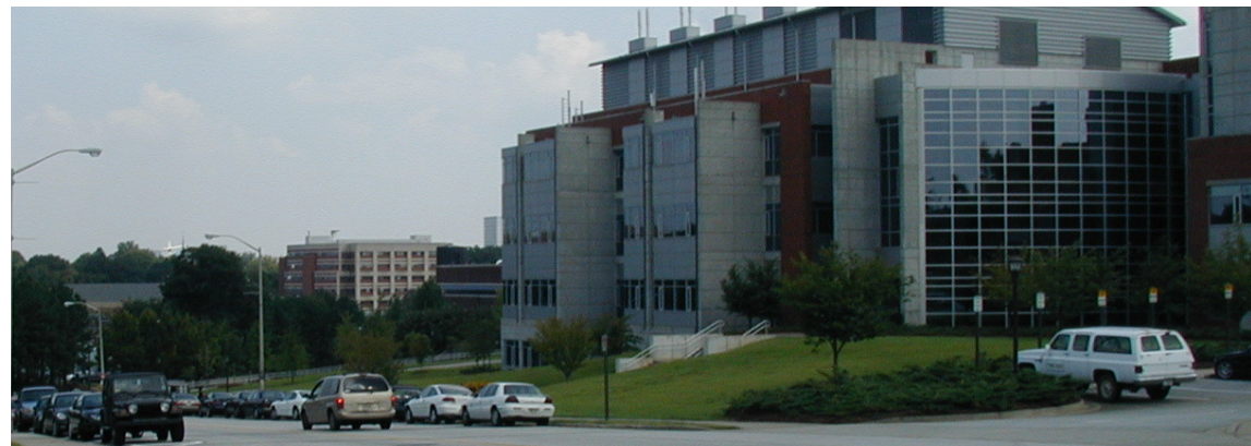
Figure 5-30: The bold architecture of the J. Erskine Love Manufacturing Building and other buildings along Ferst are signatures for the Ferst Fifth corridor when set within a landscape of natural plant communities.
