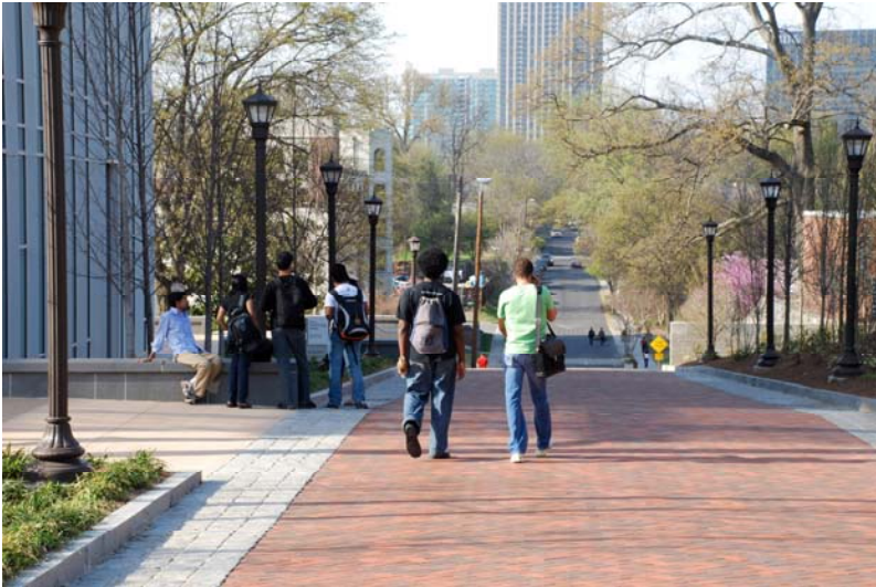
Figure 6-30. Atlantic Promenade north of Ferst, showing Pavement Type-A: Brick with granite curb and gutter
