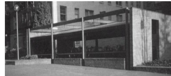
Figure 6-47: Example of Covered Long-term Parking
