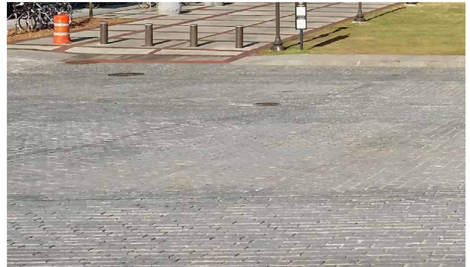
Design treatments, such as cobbles, at intersections should create safe mixing zones and slow bicycle traffic.
