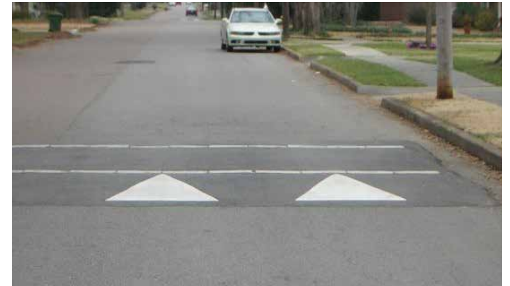
Speed humps encourage drivers to reduce speeds.
