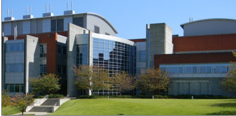
Figure 2-2: Existing Campus Facilities (Love Manufacturing Building)
