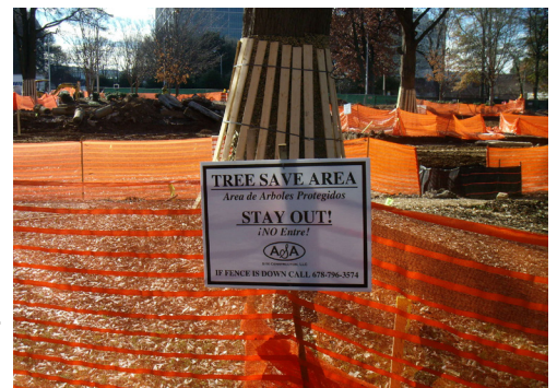
Tree protection during construction.
