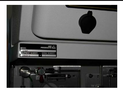
Figure 2: Equipment Commodity Code Number on an AP10 Gas Rack
