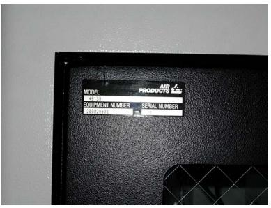
Figure 1: Equipment Commodity Code Number on an AP10 Gas Cabinet
