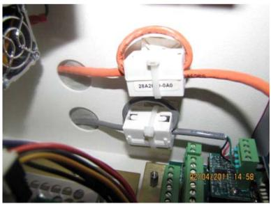
Figure 4.4b: Incoming I/O and Ethernet with ferrites installed
